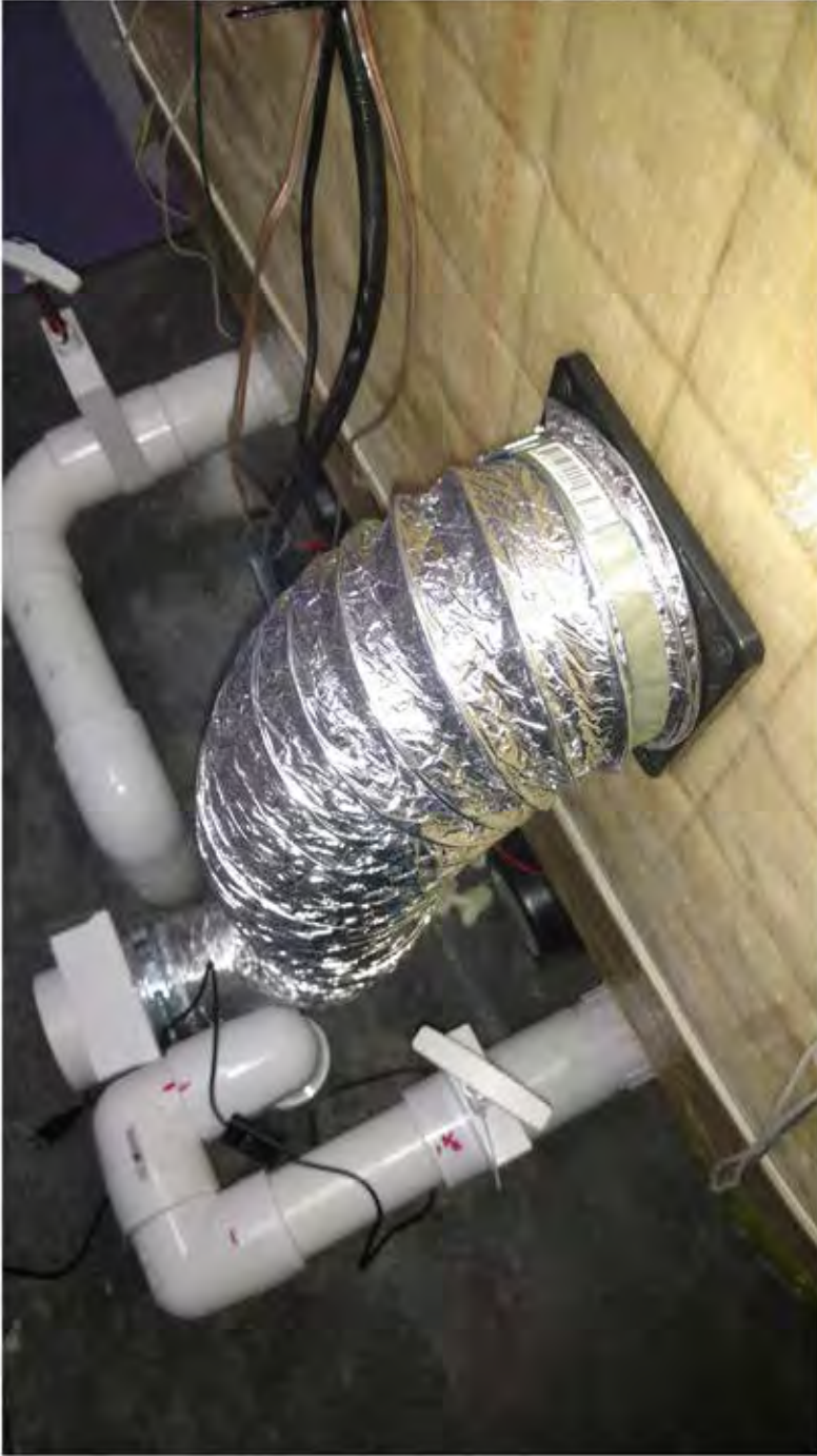
Basic blower installed on float room.
